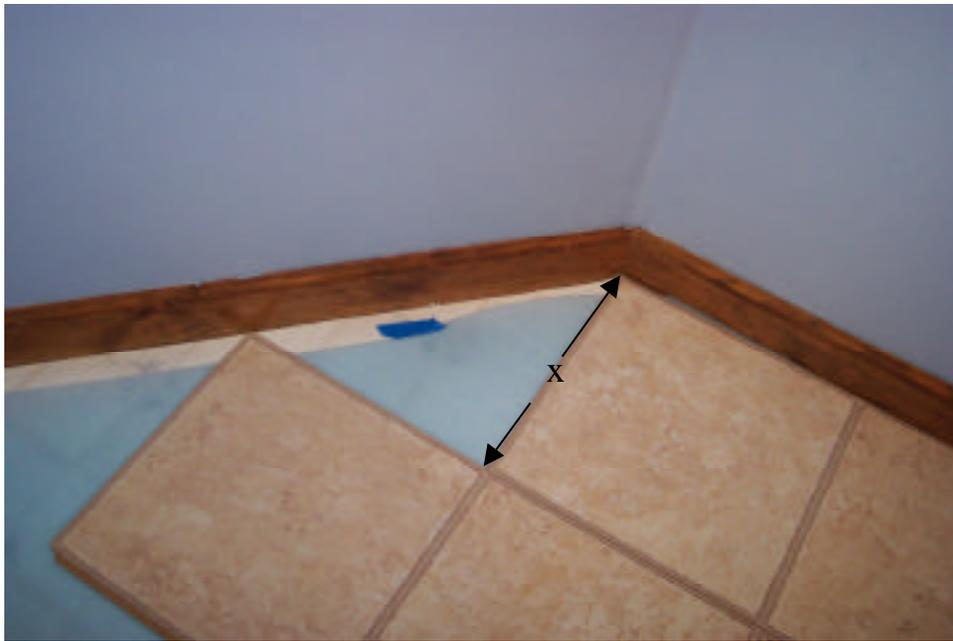
Figure 5. Measuring the starting point for the second row of laminate.
