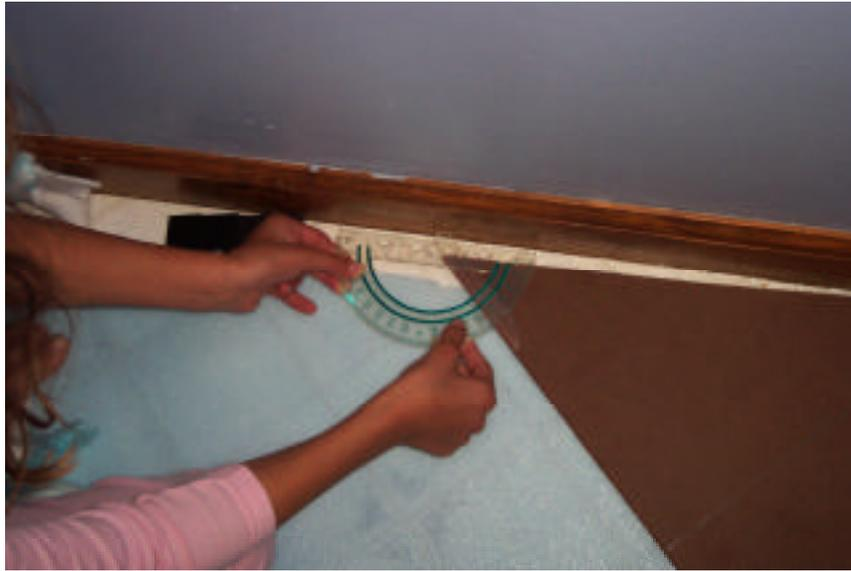
Figure 3. Measuring the congruent angle at a spot where the wall is straight.
